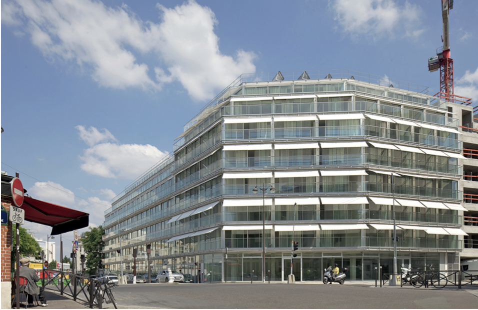
Façade principale [source: architecte]
